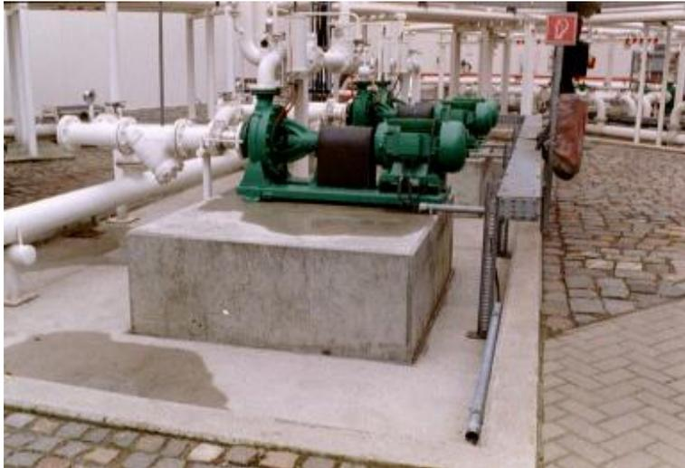
*Delivery pumps for fuel and heating oil in a pump basin:*
