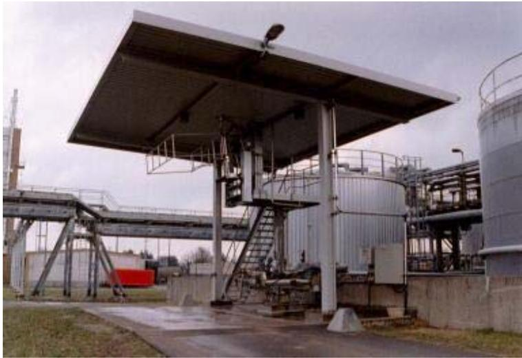
*Road tanker station used for loading and unloading tank cars:*
