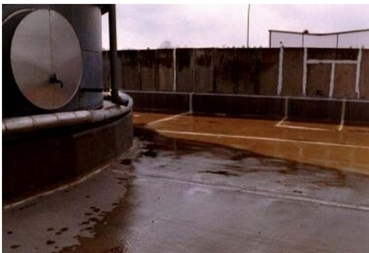
*Flat bottom tank in a renovated secondary containment:*
