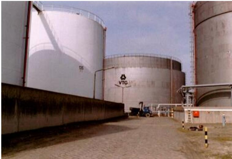
*Flat bottom tanks in secondary containment:*
